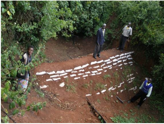
Figure 17. The dam to store water built with "Do-nou" (Kenya)
